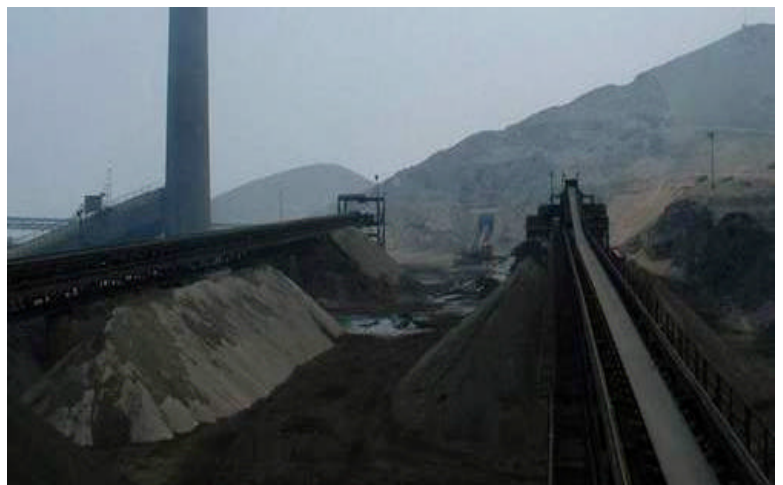
Figure 2: Southern Peru Site
