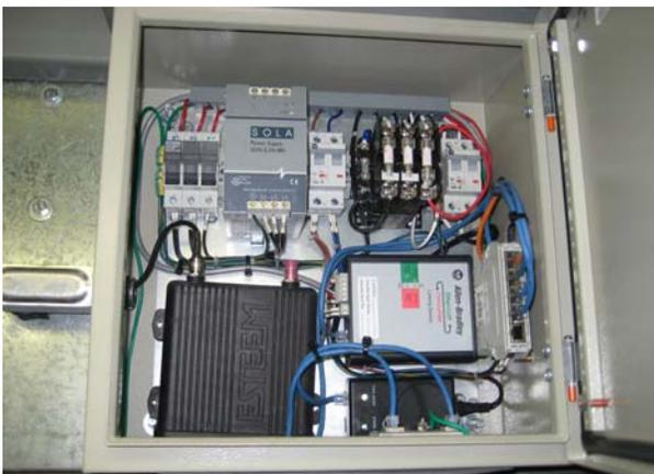
Figure 1: Rockwell DeviceNet to Ethernet/IP Converter
